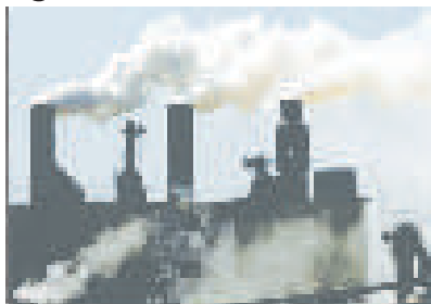
Industrial smoke Air pollution
